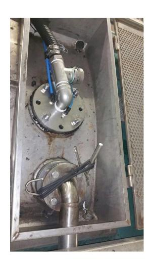
Pneumatic pressure sensors in control cabinet (below). Pneumatic hoses from tank wall to cabinet.
